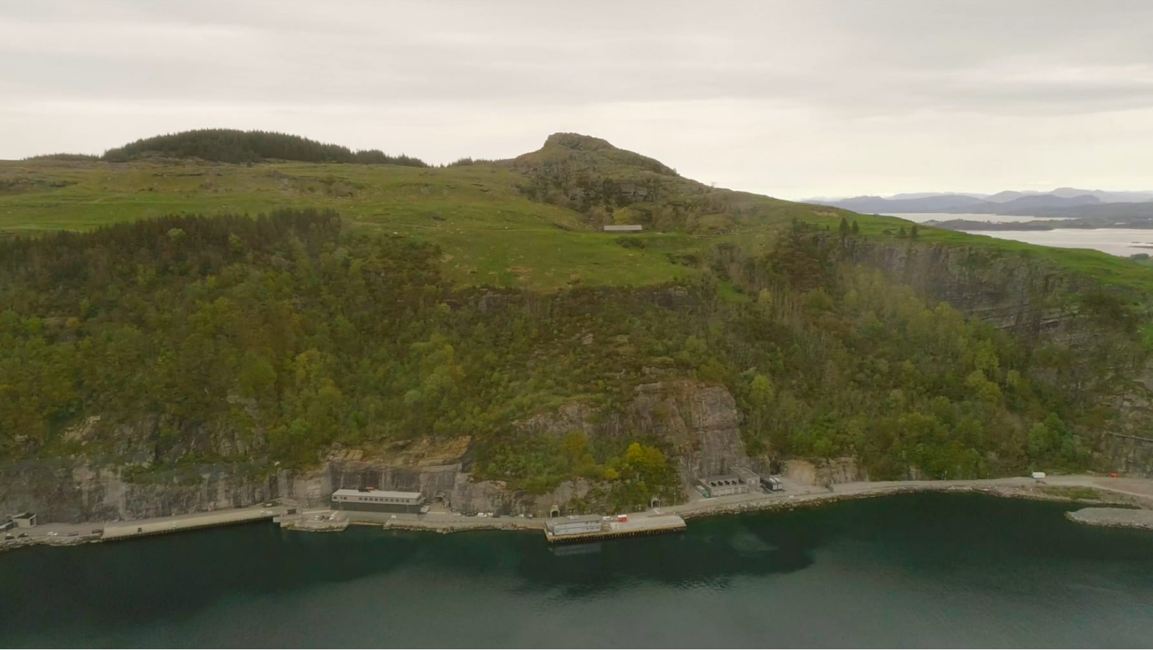
Green Mountain's DC1-Stavanger site - A mountain hall facility
