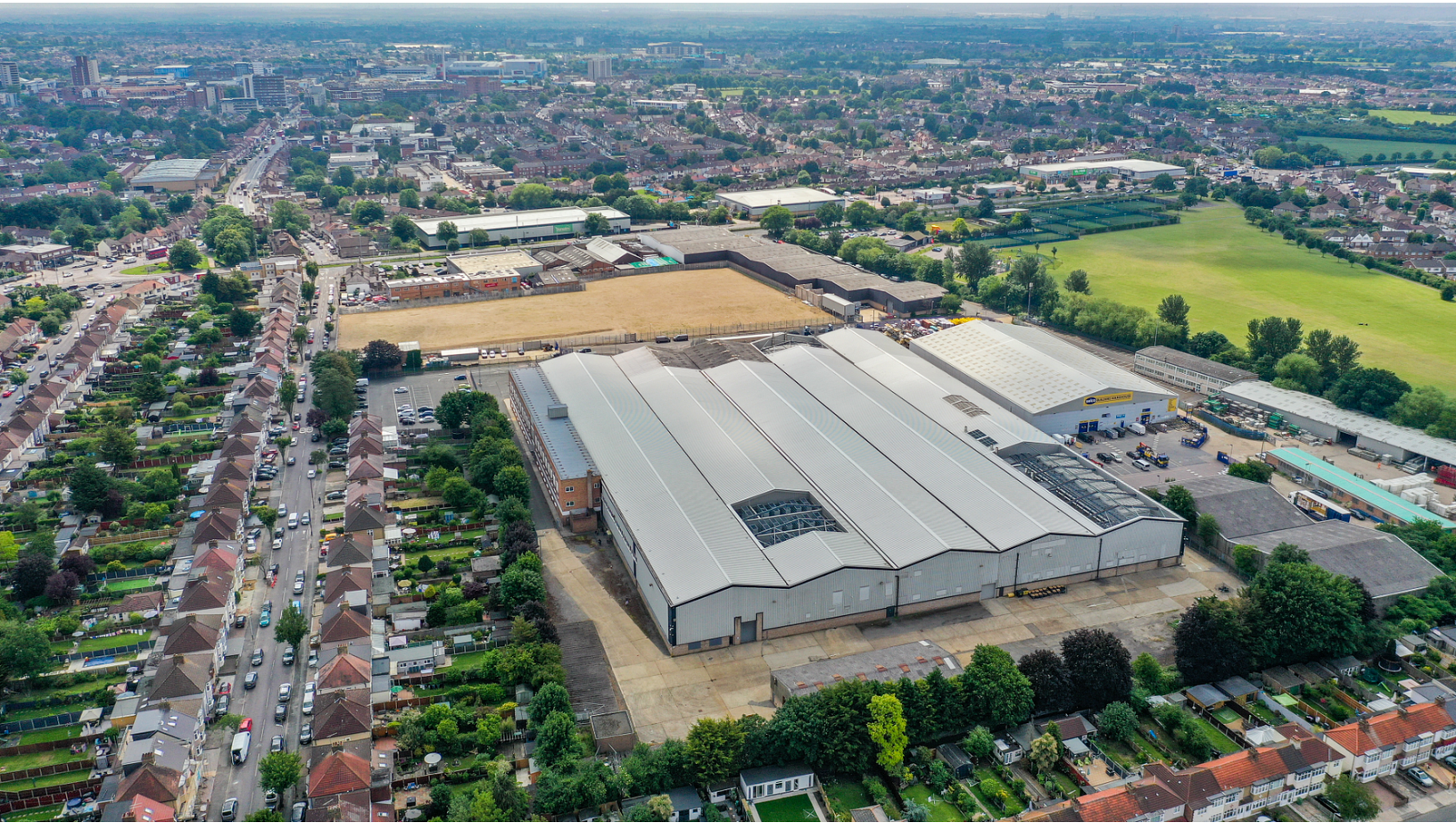
Aerial view of the LON1-East Data Center Campus.
