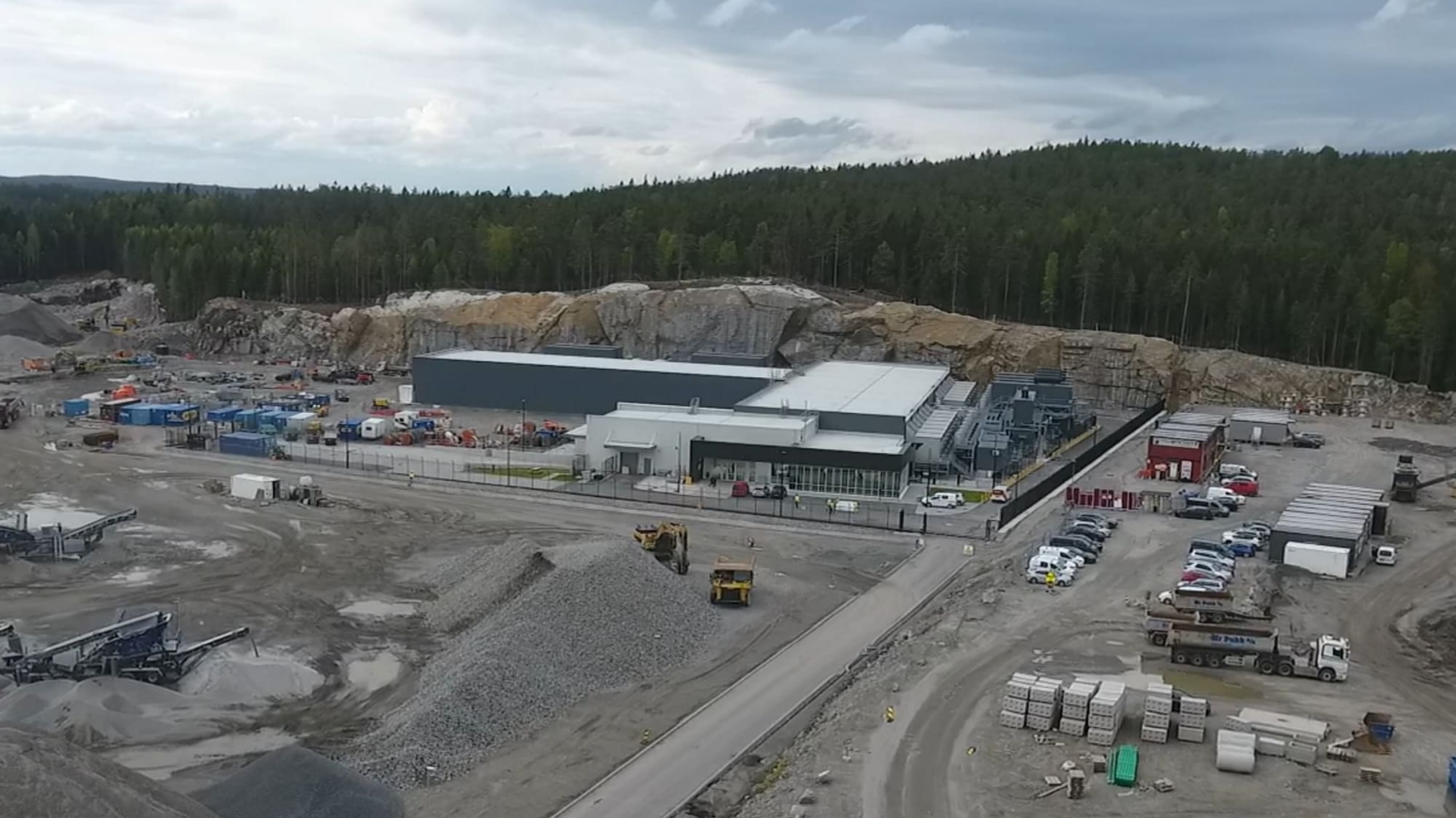
Busy work at the construction site of the DC3-Oslo expansion.
